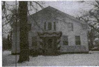
The Leland house, 3850 North Territorial Road, Northfield township, is an unusually wide five-bay gable front example.
